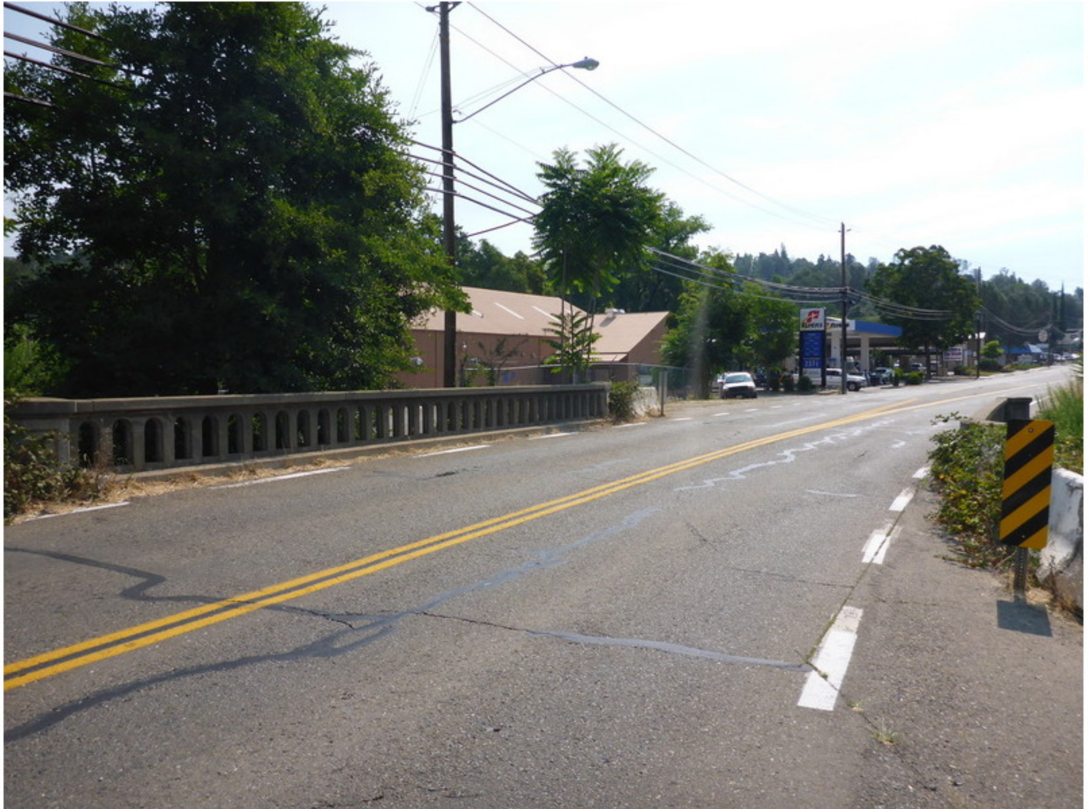
Photo No. 1 Routine roadway looking east
